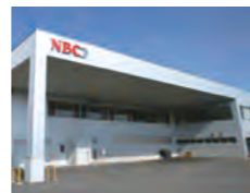
Shizuoka Kikugawa Factory
